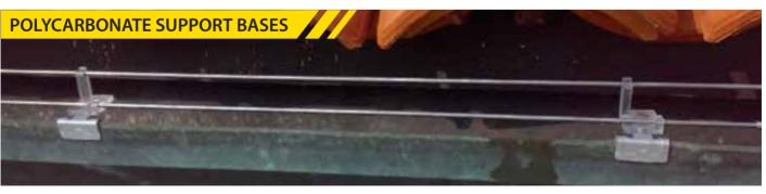
Position one base Mod. 420 every 33 cm in case of pigeons and one every 25 cm in presence of seagulls. Remember to install the lower part of the base outwards, facing the direction where birds come from.
