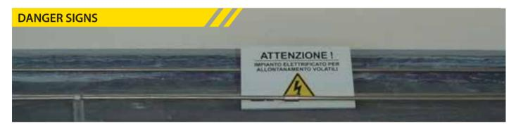
It is recommended to put some danger signs along the line for signalling its presence. They are available in Italian, English, French and Spanish. They are not required by law in Italy, yet they represent a useful device to avoid accidental contact with the electric line.
