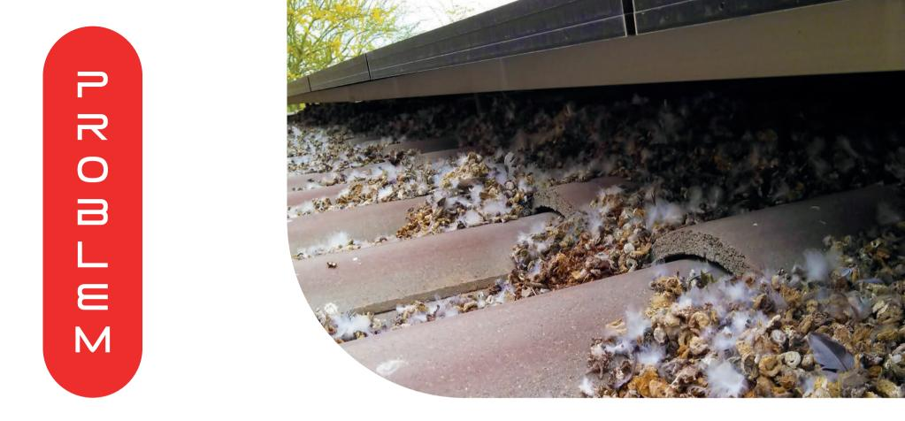
The roof of houses is usually an interesting refuge for pigeons attracted by heat loss through the roof and chimneys. In the case of roofs with photovoltaic systems, the heat accumulated during the day by the panels through solar radiation provides additional comfort and shelter for pigeons, which tend to inhabit the roof even in winter.
